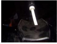
4. Attach the adaptor supplied and join to existing the hose from the water valve
