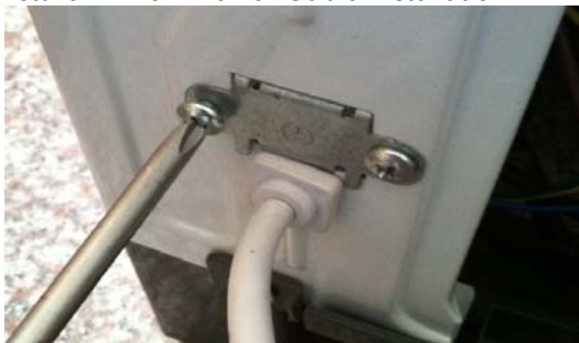
Picture 14.49 Power Cable installation - 2
