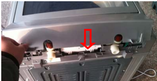
Picture 14.2 Rear panel installation - 1
